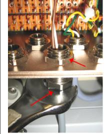
6. Tighten the nut with a wrench to secure in place. It may be necessary to use a second wrench to hold the top nut in place.
