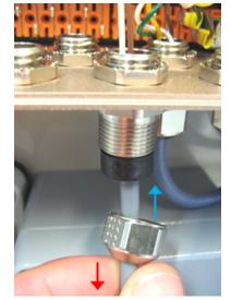
5. Pull the cable slightly with one hand until the inner shield comes into contact with the gland. Tighten the nut onto the gland with the other hand.
